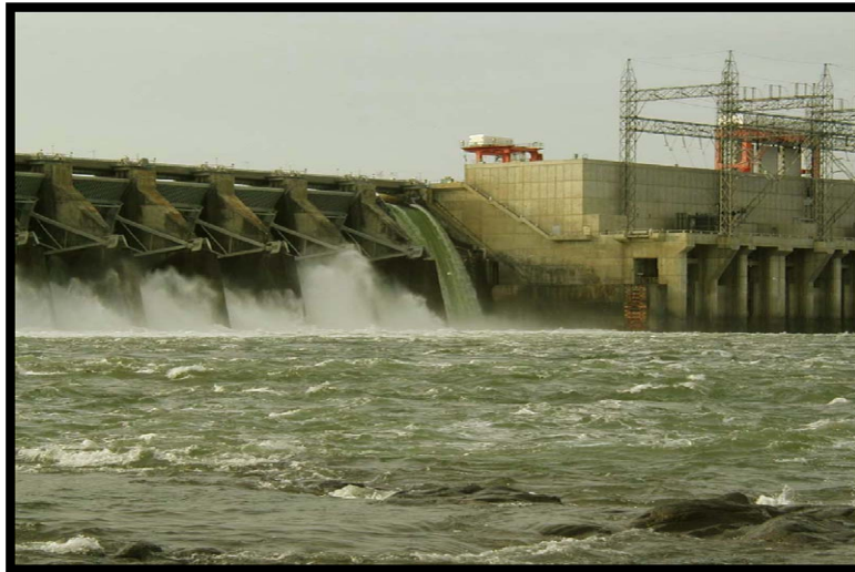
Figure 7-2. Priest Rapids Dam top spill bay 22 and standard spills at bays 17 to 21 (Corps, 2003).
