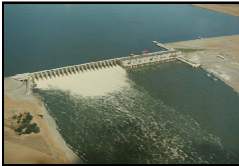
Figure 7-1. Aerated spillway flow from Priest Rapids Dam (Corps 2003).
