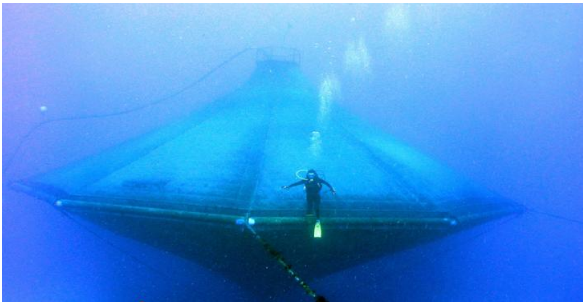
Figure 2.2.a: Submerged, “semi-rigid” fin fish enclosure in pilot OOA facility, Puerto Rico. Photo: NOAA
