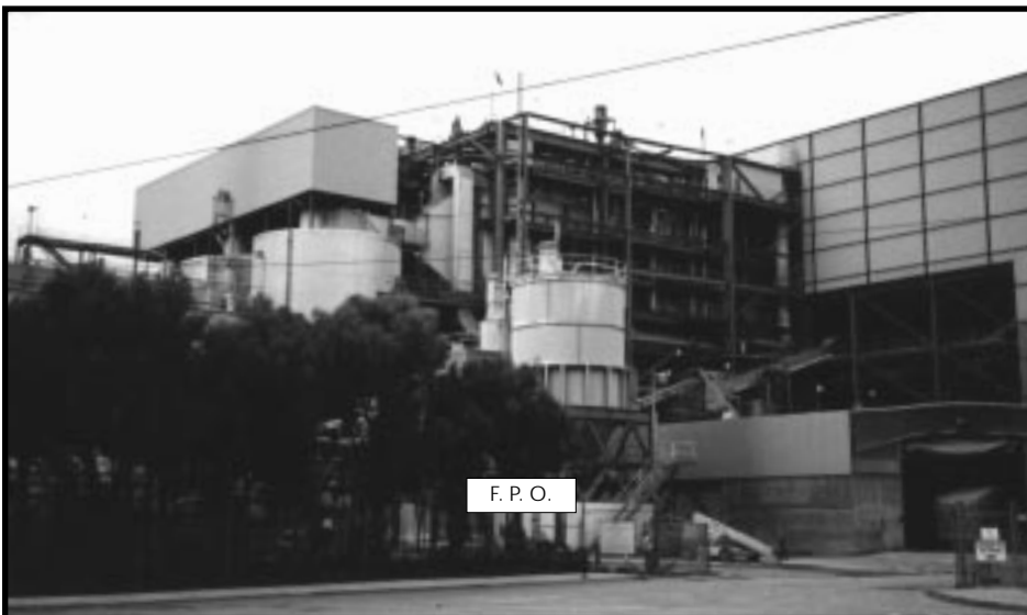
The Southeast Resource Recovery Facility in Long Beach, CA.
