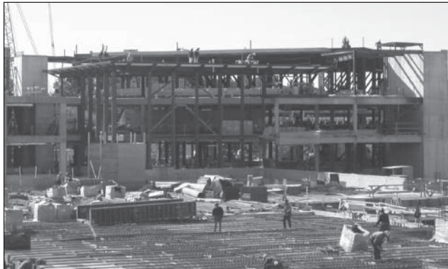
Construction of the AML Cleanroom, late Oct. 2001.
