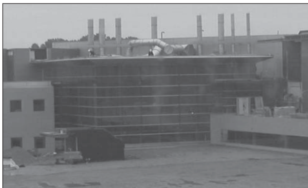
Construction of the AML Cleanroom, late Oct. 2002.
