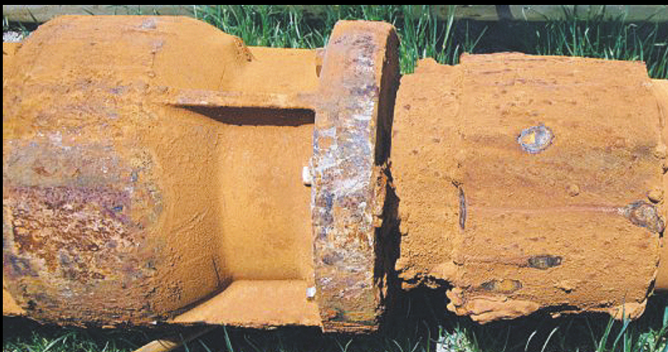
Figure 1. Encrusting material on a supply-well pump from Suffolk County, N.Y.
