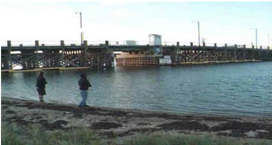
Figure 4. Beach Road Bridge.
