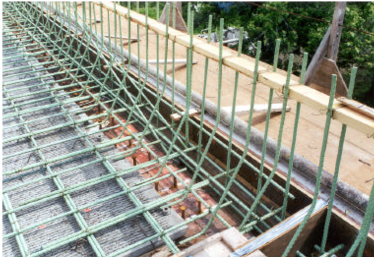
Photo 11. Inside parapet wall bars resting on plank (District 8 – Stage 1, June 24, 1999)
