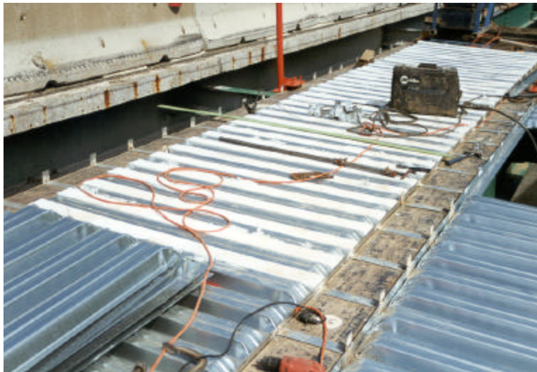
Photo 21. Polystyrene fillers in metal stay-in-place forms (District 8 – May 1999)
