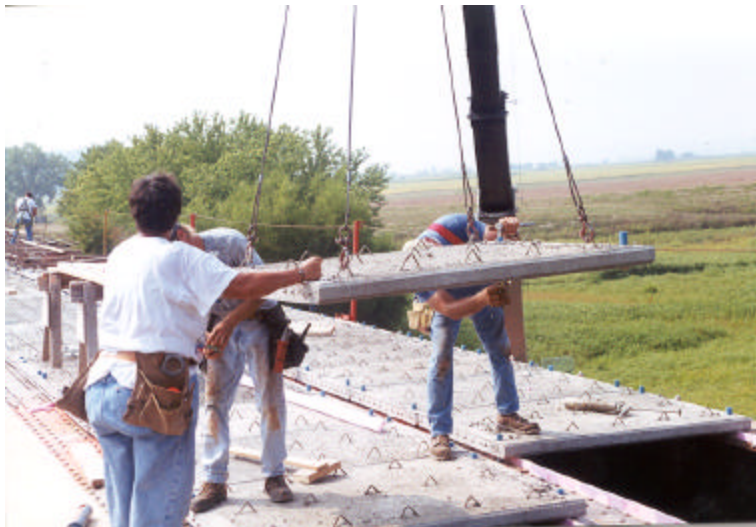
Photo 7. Deck plank seating (District 8 – Stage 2, Sept. 2, 1999)
