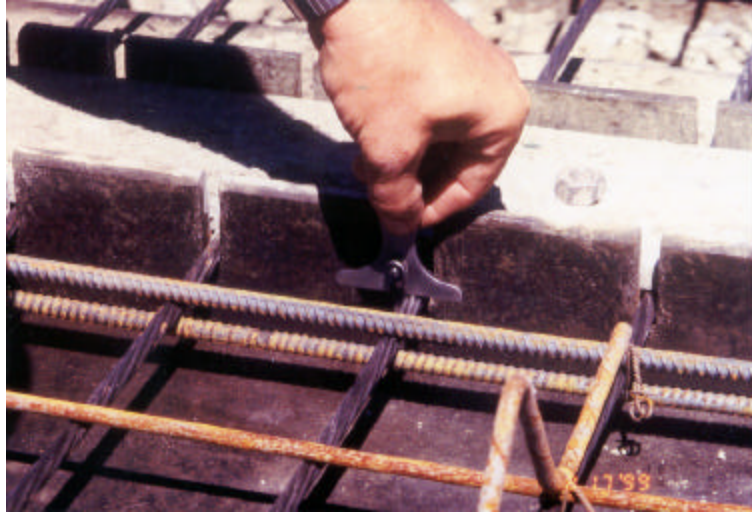
Photo 3. Checking vertical location of strand with micrometer
