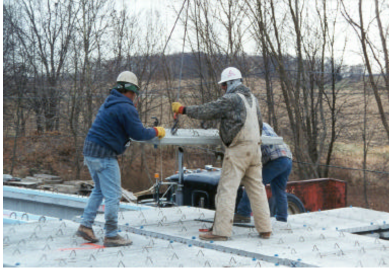
Photo 9. Deck plank seating (District 6 – Stage 2, Dec. 1, 1999)
