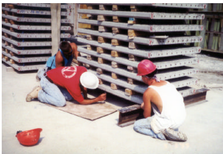
Photo 6. Checking deflection with stringline
