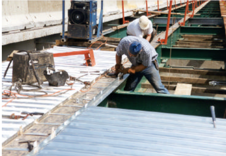
Photo 20. Seating metal stay-in-place forms (District 8 – May 1999)
