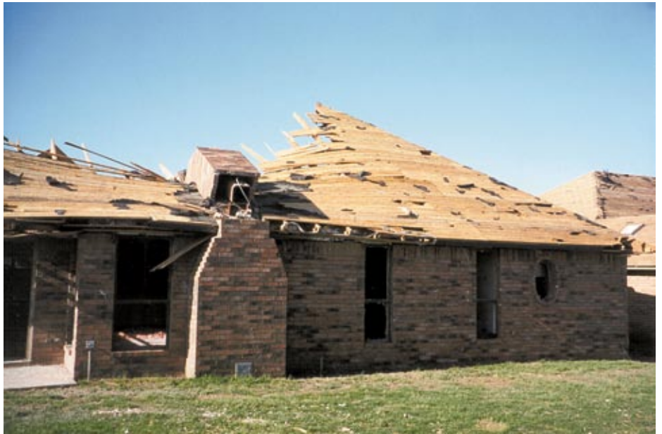
Avoid selecting a refuge area that is near a masonry chimney (Moore, OK).
