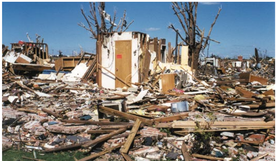
View of remnants of an interior room of a house that survived a strong tornado.
