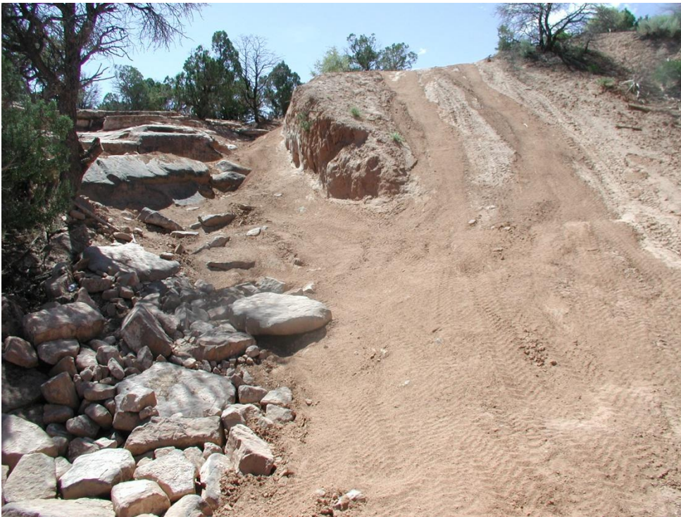
Photo 2: Ingress and Egress Point to Access Channel Route in Sub-Region E, Showing Signs of Accelerated Erosion and Fine Material on Surface Likely to be Mobilized During Next Runoff Event
