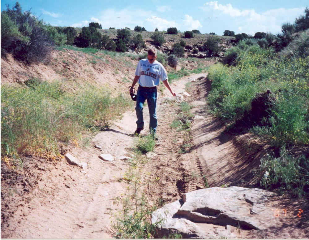
Photo 1: Route in Ephemeral Wash in Sub-Region E, Showing Pulverized Channel Substrate, Ready for Mobilization with next Runoff Event.
