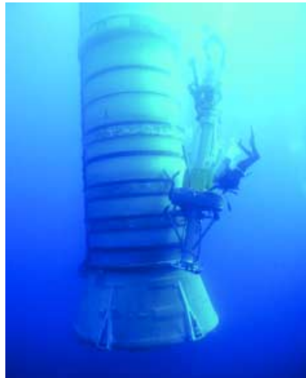
Divers installing EDOP.
