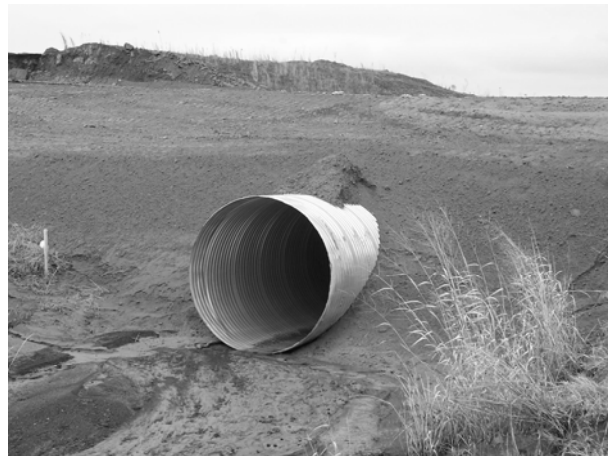
Figure 6. Sixty-six inch culvert bedded in and backfilled with ash.
