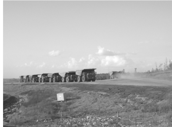
Figure 5. Haul truck fleet parking area constructed with ash.
