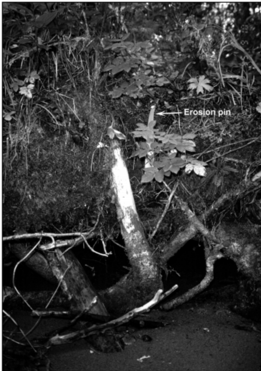
Figure 17. Undercut below erosion pin at RW's Campground study site, September 10, 1996.
