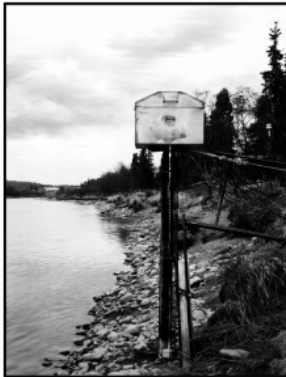
Figure 7. Wake gage instrumentation (A), example of wake record (B), and typical installation adjacent to streambank (C).
