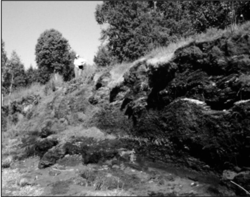
Figure 14. Slump of cohesive bank material at the Cunningham Park study site, July 31, 1996.
