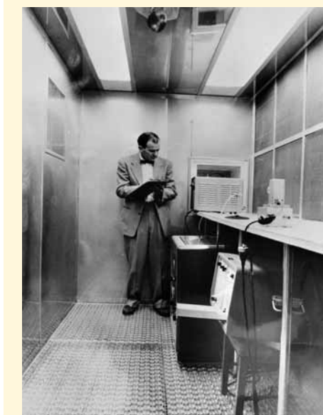
WHEN WILLIS WHITFIELD came up with the idea for the laminar airflow clean room, it was intended to provide a dust-free environment for close-tolerance weapons parts. Little did he — or anyone else — know that his idea would become a basic enabling technology for the $1.2 trillion microelectronics industry. Willis is seen in the photo above monitoring air quality in an early clean room. A page from his laboratory notebook, at right, shows a cross-section of the proposed clean room design.
