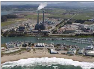
The power plant in Moss Landing contains a seawater distillation plant that produces fresh water for use in the power production process. Photo: NOAA/MBNMS
