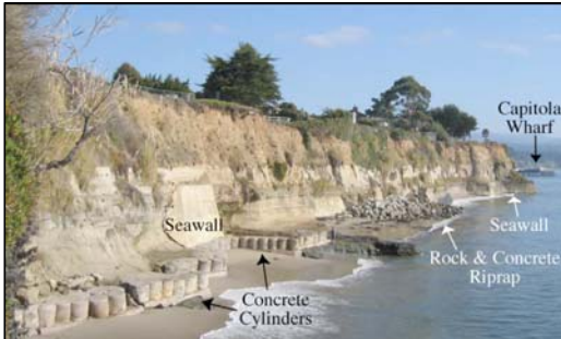
An unplanned assemblage of coastal armoring structures at Opal Cliffs near the city of Capitola (on the north side of Monterey Bay). Photo: R. Stanski, MBNMS/NOAA/SIMoN
