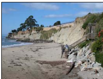
Exposed cliffs are reinforced to slow erosion caused by wave action. Photo: NOAA/MBNMS
