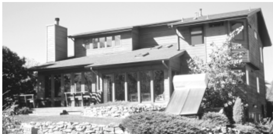
An example of an energy-efficient home in a cold climate using direct-gain passive solar heating.
