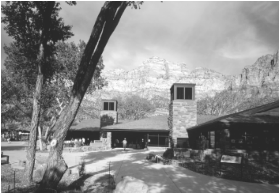
The Zion Visitor Center is designed to use 70% less energy than a typical building without costing more to build.
