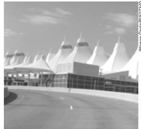
Denver International Airport in Denver, Colorado, is an example of a fabric-covered roof.
