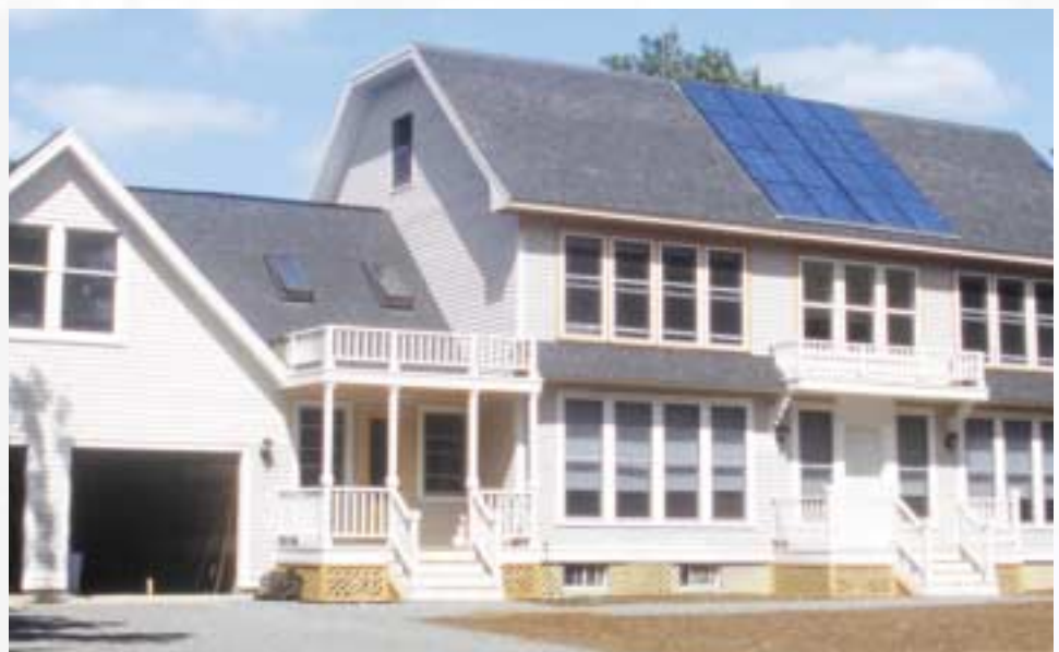
Solar energy meets 78% of this home's heating needs. The 16 PV modules, which can be factory-installed or site-mounted on the roof, provide virtually all of the home's electricity. (Manufacturer: AvisAmerica homes.)
