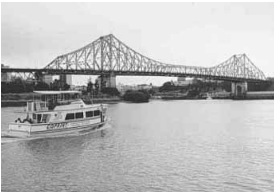
Figure 6. Bridge with no instream sections. Brisbane, Queensland (Photo courtesy Main Roads Photo Visual Library).
