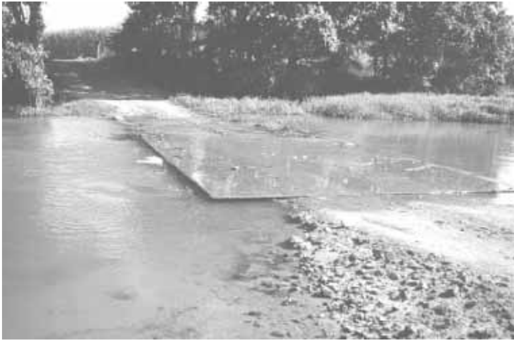
Figure 17. Low-level crossing with low-flow culverts. Tully, Queensland.
