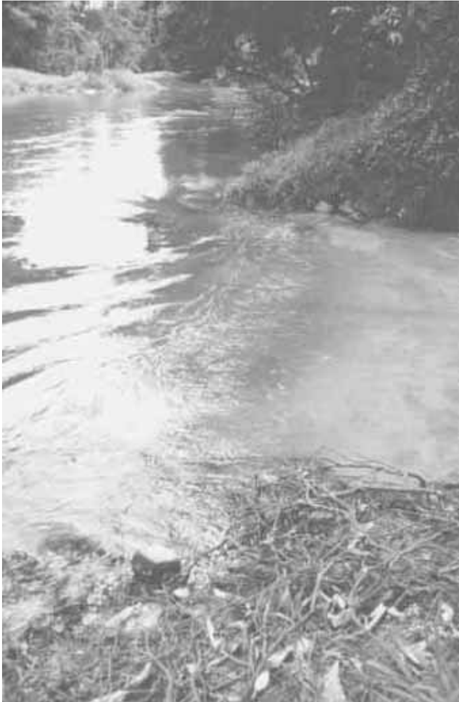
Figure 21. Slow water areas can be created at the edges of low-level crossings by extending the stream banks into the stream to create an 'inlet'. Tully, Queensland.
