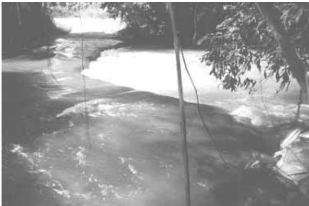
Figure 18. Concreting of low-level crossings can result in a drop on the downstream side that is impassable to fish. Murray River, north Queensland.
