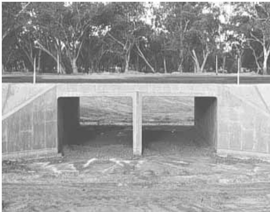
Figure 12. Short, wide culverts allow for maximum culvert illumination (Photo courtesy Main Roads Photo Visual Library).
