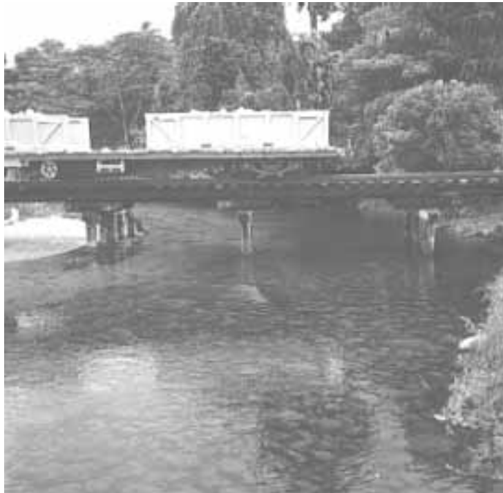
Figure 9. Irregularities in the bed and banks of natural streams create slow water areas that allow fish passage (Photo courtesy A. Hogan).
