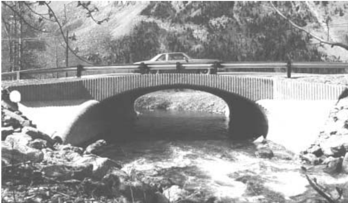
Figure 8. Bottomless arch culvert (Photo courtesy R. Pritchard).
