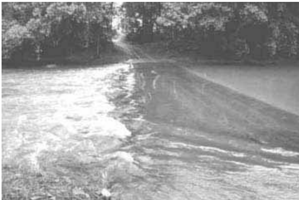
Figure 20. Concreted rocks and boulders can create a turbulence barrier to migrating fish. Tully, Queensland (Photo courtesy A. Hogan).
