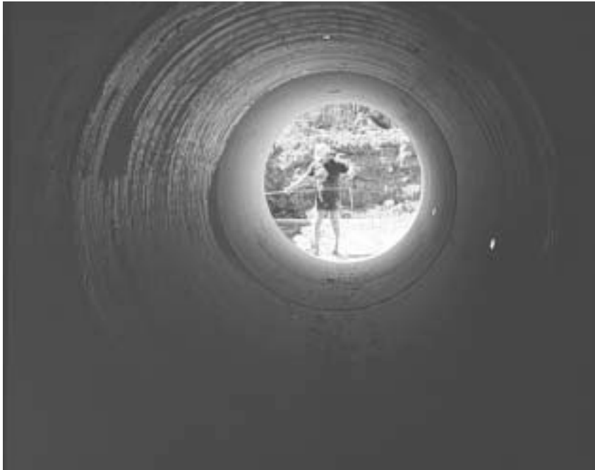
Figure 13. Long culverts are dark (Photo courtesy Main Roads Photo Visual Library).
