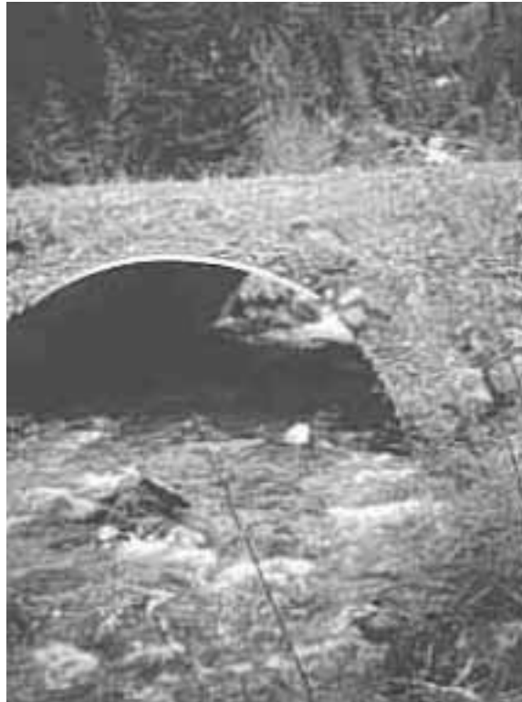
Figure 5. Culverts can be countersunk below stream bed to prevent perching (Photo courtesy K. Bates).
