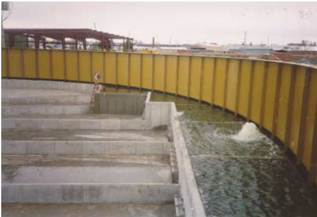
Figure 6-10. Cheboygan - Photographs of Circular CSO Storage Tank
