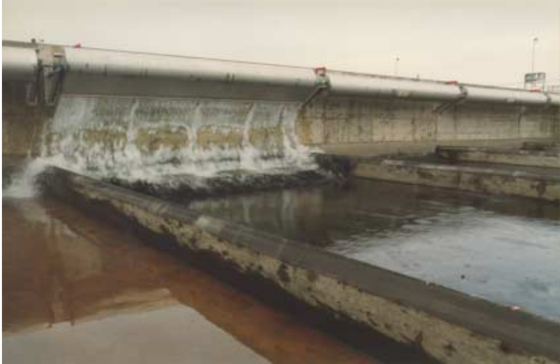
Figure 6-20a. 14 th Street Pumping Station - Flushing and Sequence for Tank B4
