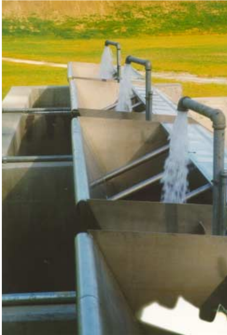
Figure 6-17b. Wheeler Avenue - Photographs of Filling Tipping Flushers and Overall CSO Storage Tank
