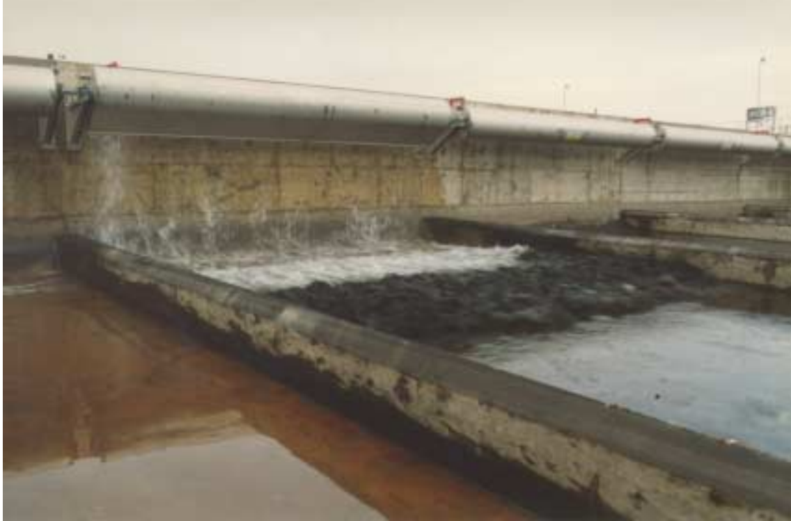
Figure 6-20c. 14 th Street Pumping Station - Flushing and Sequence for Tank B4
