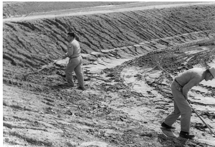
1930's Pond Construction
