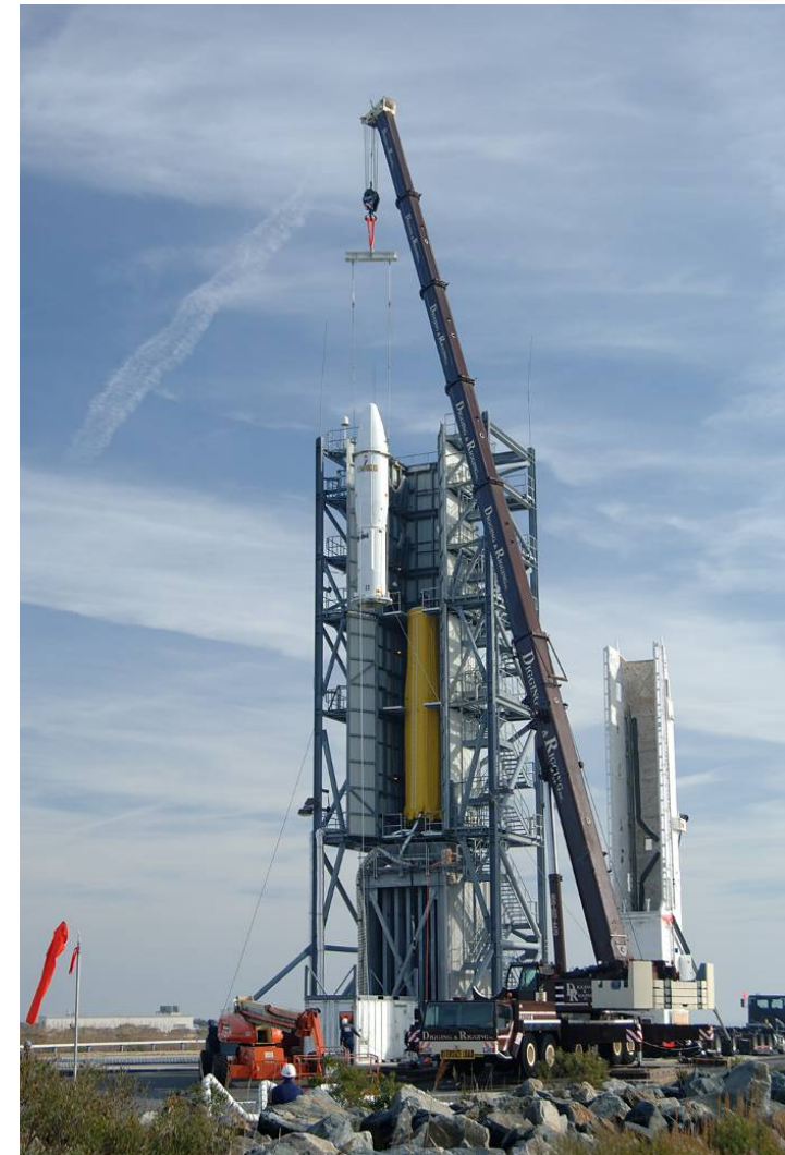
Upper Stack Emplacement on 11/28/06
