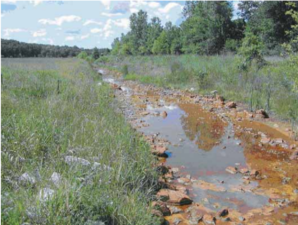
Figure 7. Acidic mine drainage in an open limestone channel downstream from the Huntsville Gob reclamation project looking north from sampling site HG-7S.
