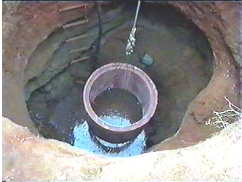
Figure 3: Set up of RCC rings into Kararo HDW
