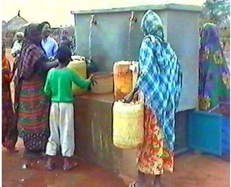
Figure 2: Gobicha water point
