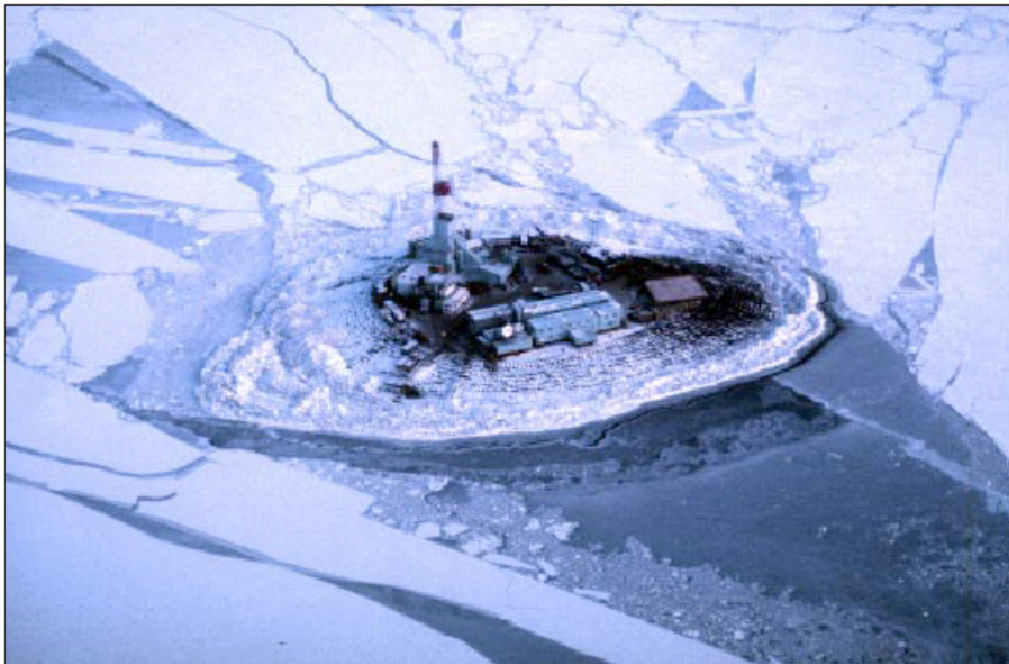
Figure 2-4: Freeze-up around Seal Island in the Alaskan Beaufort in mid-October with moving young ice. The open wake created by the island is covered in a mix of grease and nilas in the center and brash packed into the edges of the lead (Vaudrey, 2000)
