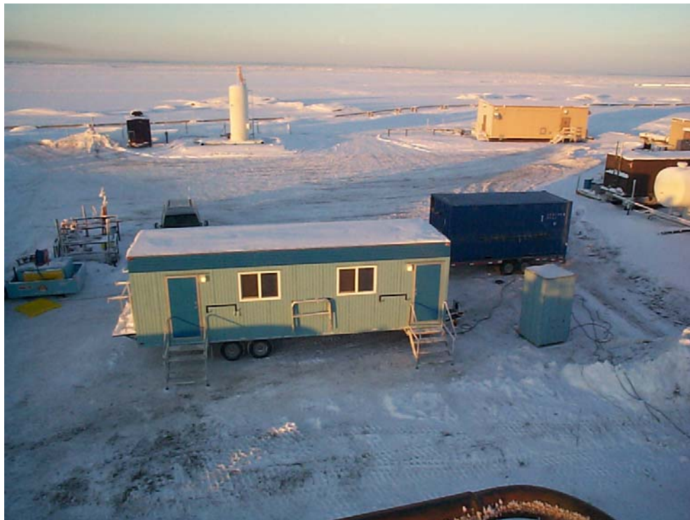
Figure 4-8: Warm-up trailer and portable diesel generator.
