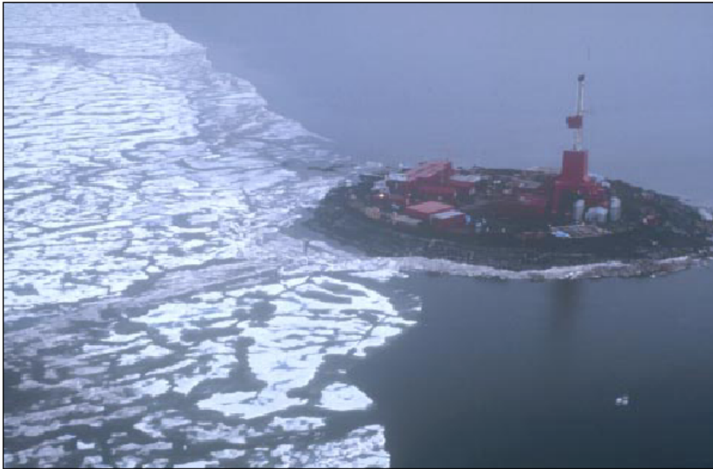
Figure 2-3: Break-up conditions around Seal Island in the Alaskan Beaufort on July 8, 1985 (Vaudrey, 2000)
