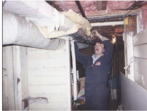
Installing Duct Wrap
