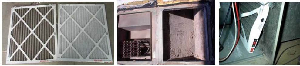
These illustrations show dirty and clean pleated filters, a very dirty coil that had been exposed to unfiltered air and a poorly installed filter that leads to filter bypass and most of the air flowing through this system would be unfiltered.
