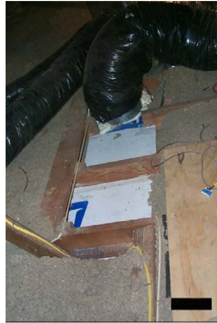
Envelope sealing: Often there are large building cavities or chases that are open to outside via attics, crawlspaces or garages. This is an example of a sealed chase viewed from the attic. The large white rectangles are duct board insulation that has been used to block off large open areas
