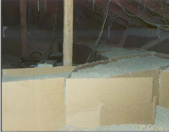
Blown –in insulation with cardboard forms
