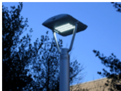
Figure 1. Several HPS fixtures (left) were replaced with LED pole-top mounted luminaires (right) to illuminate a pedestrian area at a Federal Aviation Administration facility in Atlantic City, NJ. A full report on this installation is available at www.netl.doe.gov/ssl .
