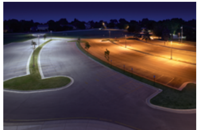
Figure 2. Installation of LED parking lot lights (left) compared to HPS lights (right) shows the difference in color appearance and distribution. Photo credit: Beta Lighting.
