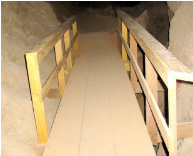
New railings have recently been installed on existing wooden structures in Left-Hand Tunnel. (NPS Photo by Tom Bemis)
