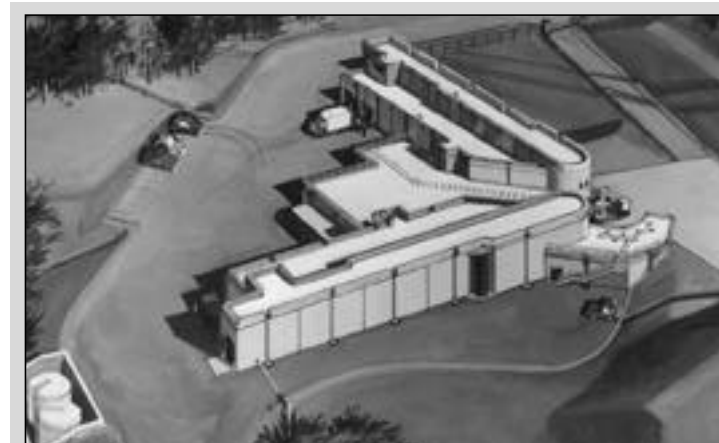
DARHT. The Dual-Axis Radiographic HydroTest Facility will produce high-energy beams from two accelerators to create three-dimensional images of the behavior of materials under explosive conditions. The facility is expected to be operating in about five years.
