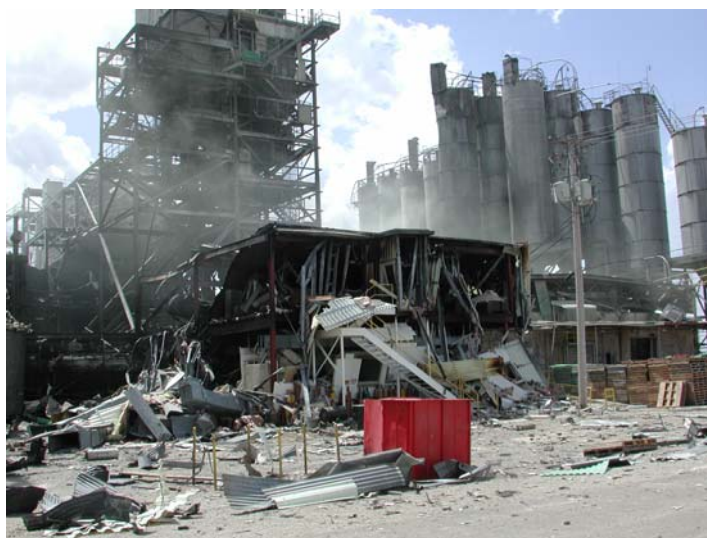
Figure 5. Damage to the Safety and Engineering offices
