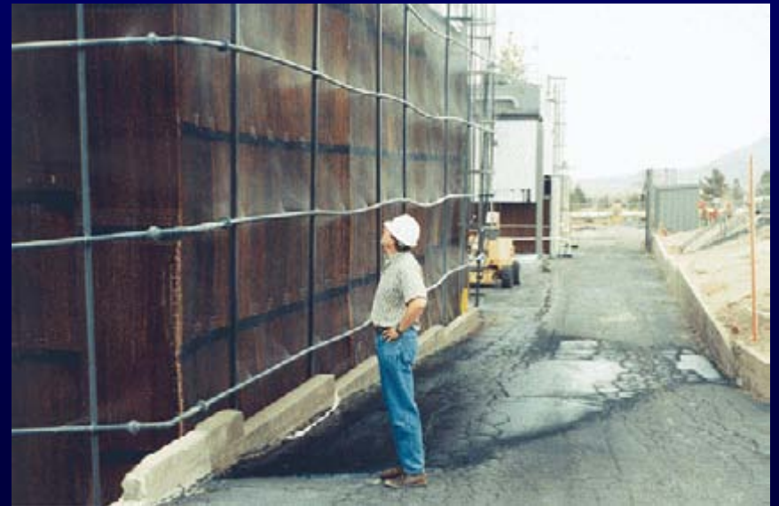
Hybrid spray/Munters system
