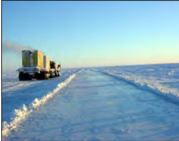
Figure 19. Rolligon with water tanks preparing to spray road.
