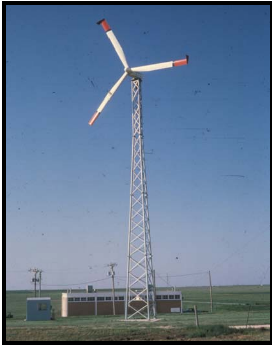
Fig. 1. The Enertech 44 was installed in 1982. The hub height was 25-m and the system supplied power to a 480 V irrigation pump connected to the utility grid.
