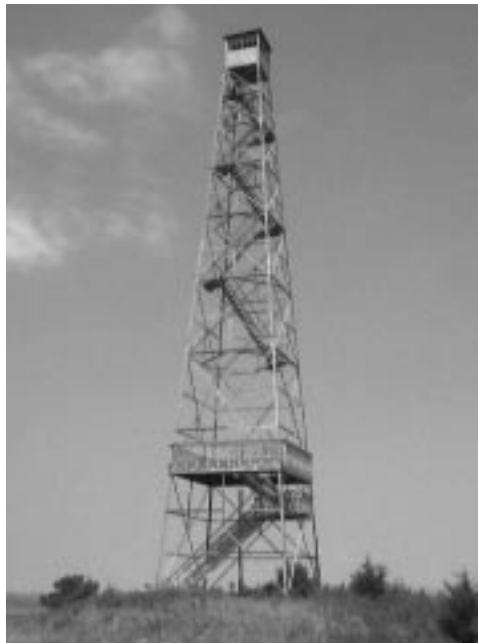
Old and new. An observation deck was recently added to the fire tower at Valentine NWR. FWS photo: Mark Lindvall.
