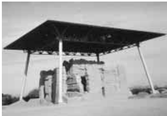
East elevation, The Great House, Casa Grande ruins.
