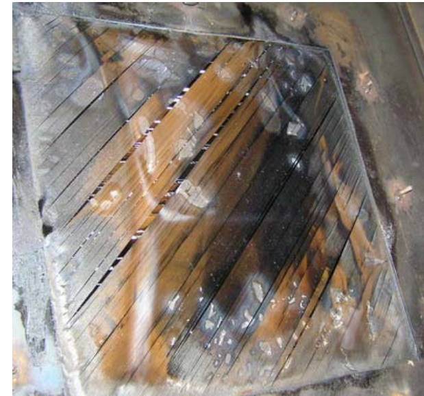
► Thermal insulation removed
