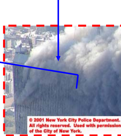
Figure 7–3. Impact damage to north and west faces of WTC 1.
