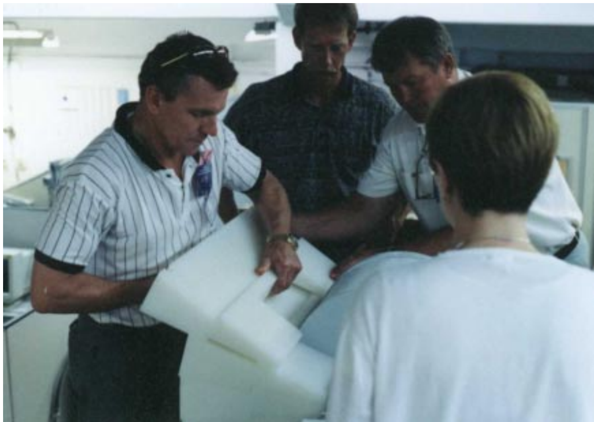
Fig. 2. UEIP and VNIITF personnel practicing for the installation of BDMS equipment.
