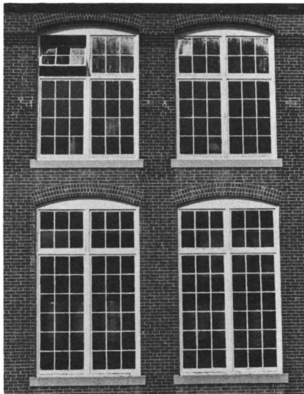
Paired windows with transoms, Lorraine Finishing Mill (1919); 603 Mineral Spring Avenue.
