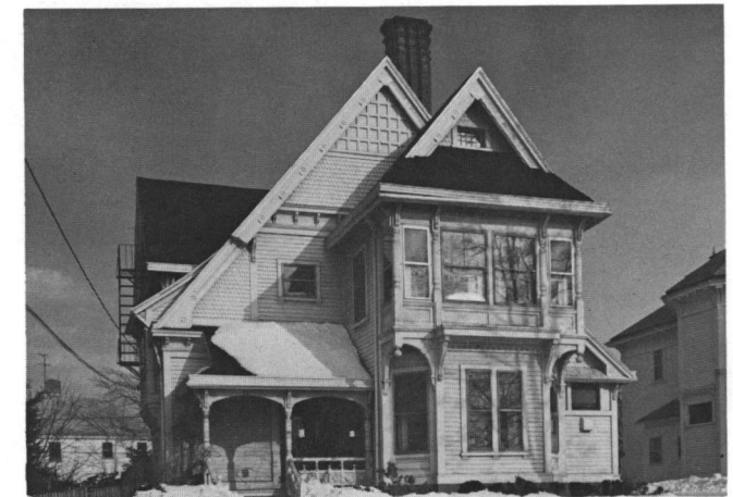
Fig. 60: Everett P. Carpenter House (1879 - 1880); 72 Summit Street; Walker & Gould, architects.
