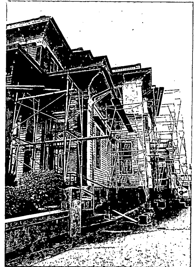
Fig. 83: Restoration of the Pitcher-Goff House, now Children's Museum (c. 1840, c. 1881); 58 Walcott Street. Exterior work funded through the Grants-in-Aid program with match provided by student labor from the W. B. Davis Vocational School.
