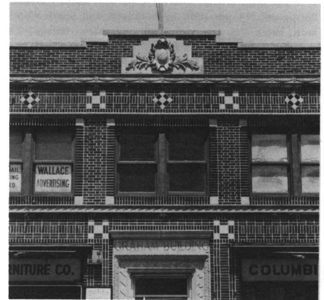
Fig. 70: Close-up, Graham Building (c. 1925); 60 Exchange Street.
