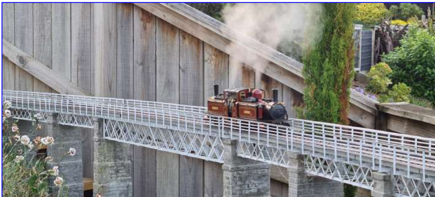
Crossing Dubh Eas Viaduct
