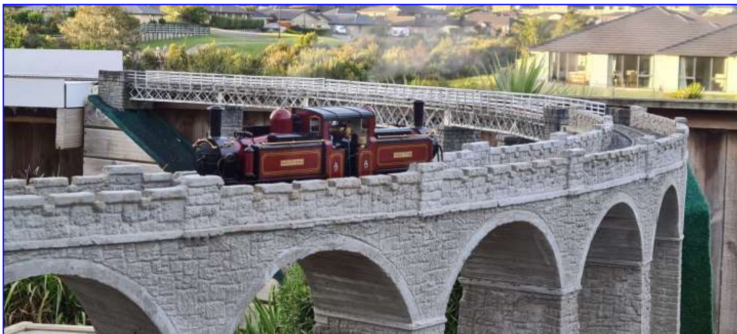
The repaired engine crossing Craigenarden Viaduct.
