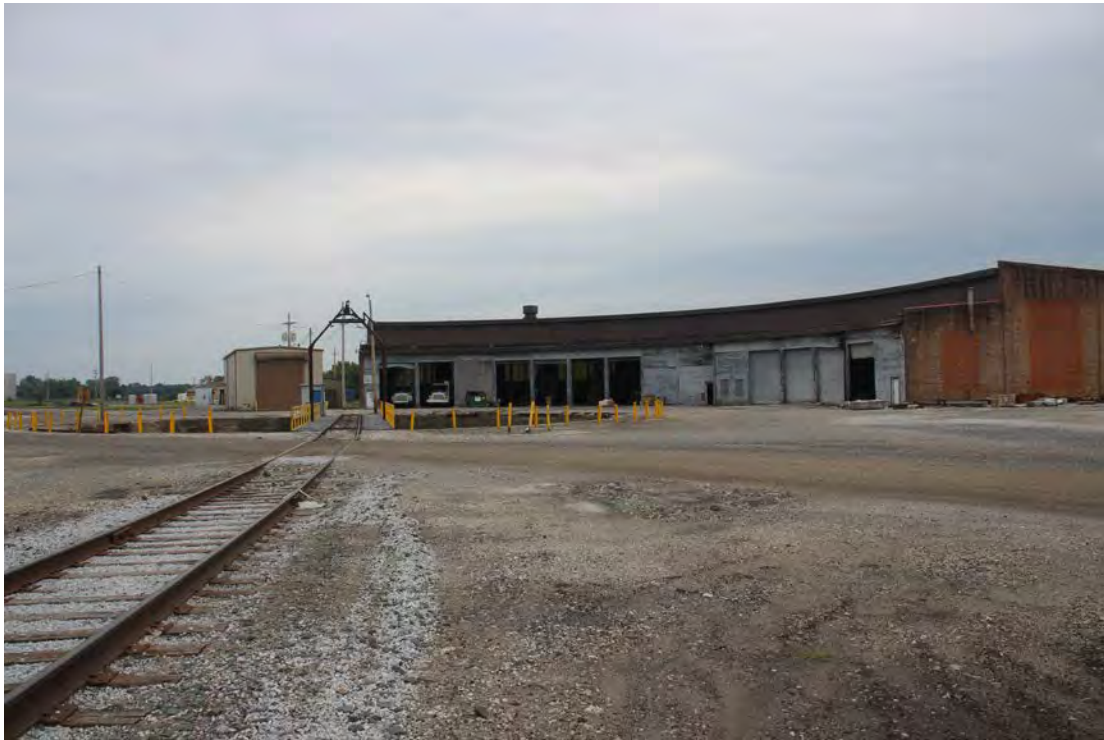
A 2017 view of the Parson Yard Roundhouse. Only 15 bays are left of which 10 can be accessed.
