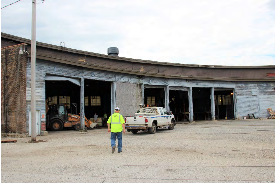
A view of bays #1 to #8. One of the MoW trucks has been pulled out and a front end loader parked in its place.
