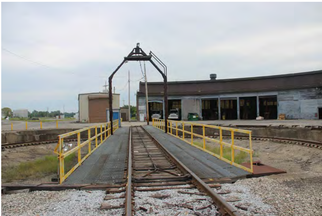
A view across the turntable toward the left edge of the roundhouse. Just to the right of the turntable is the current locomotive service building.
