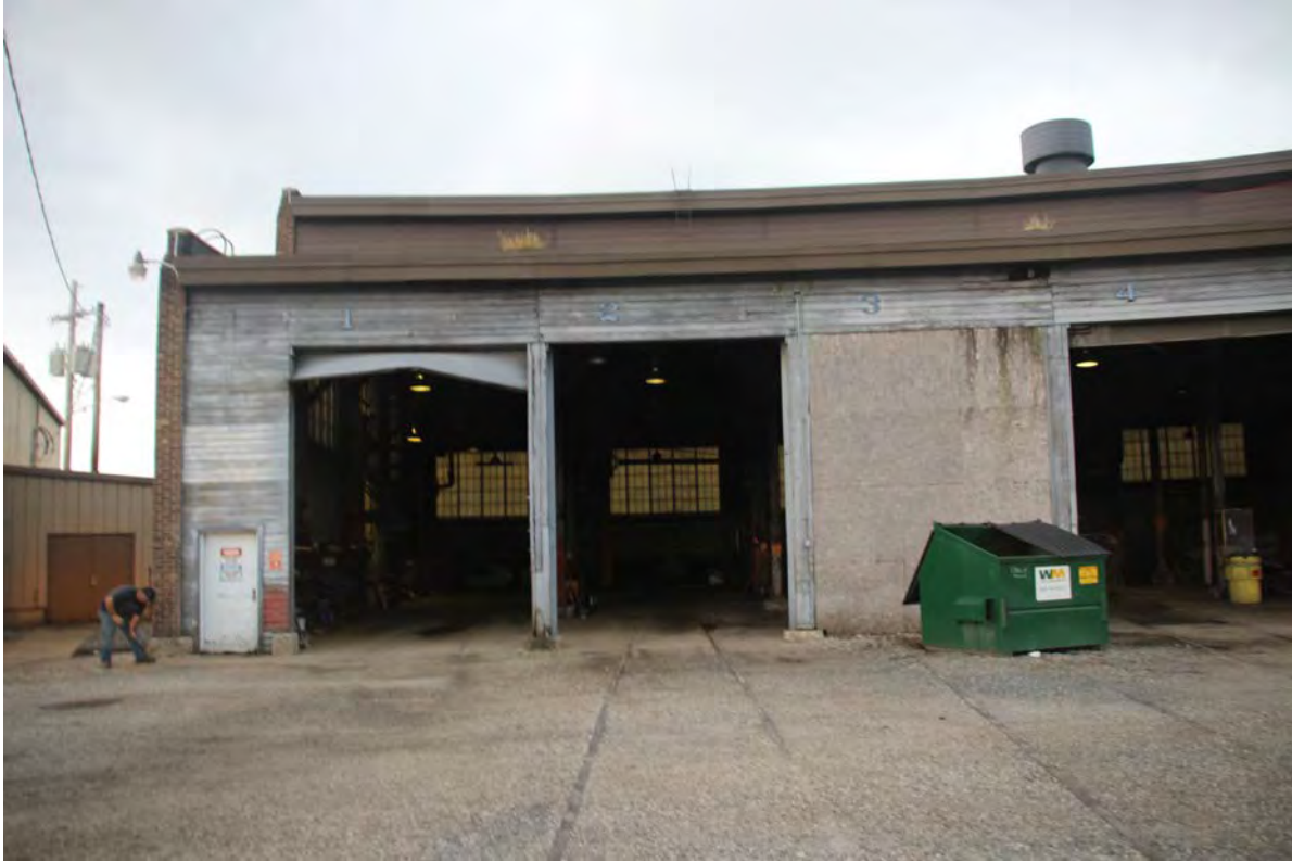
A view of bays #1 to #4. Note bay #3 is sealed.
