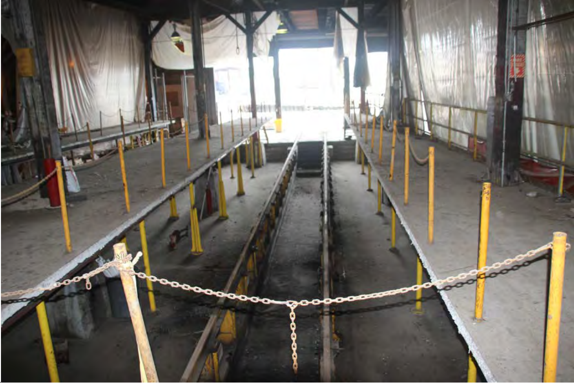
A view out from the roundhouse from inspection bay #8
