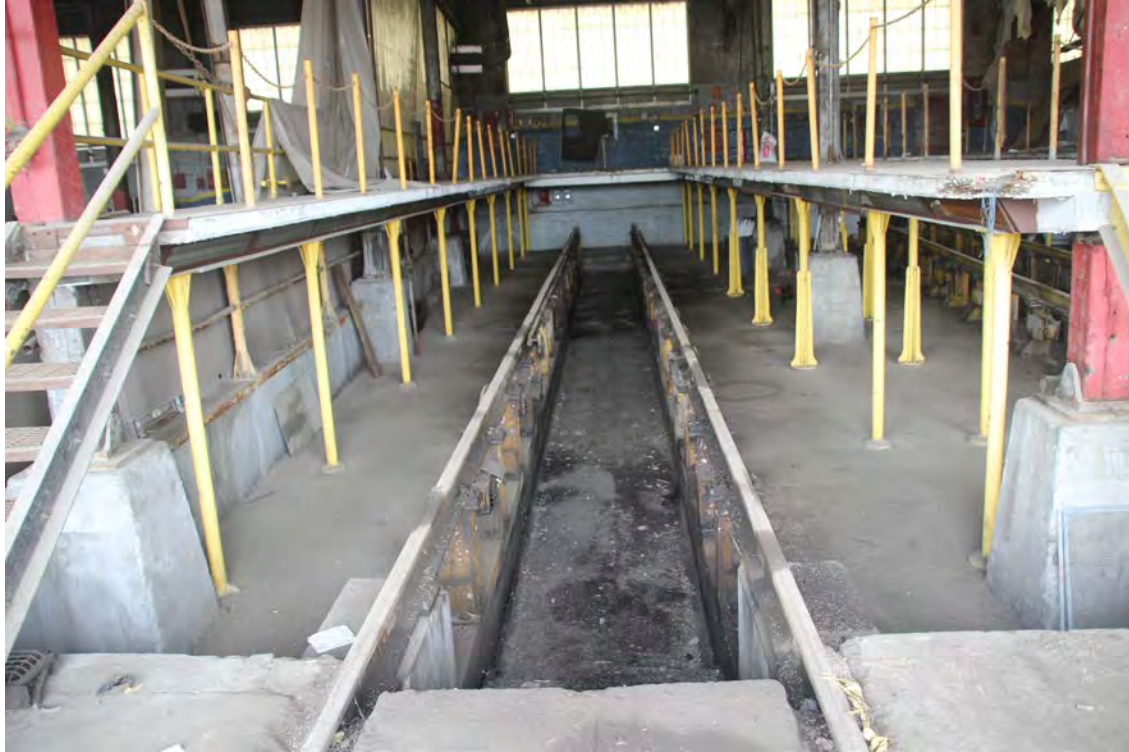
A view into bay #14. Note that the inspection pit is still in place.
