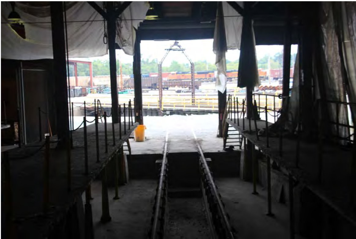
A view from bay #14 looking out to the turntable. Plastic sheeting was to protect workers from pigeon droppings and hold in heat.
