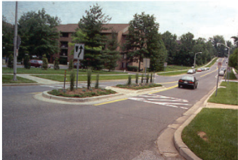
Median Refuge Near Intersection
