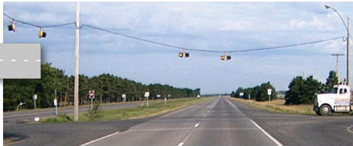
Warning Flashers at Rural Intersection, Minnesota Department of Transportation Final Report No. 1996-01. 1997
