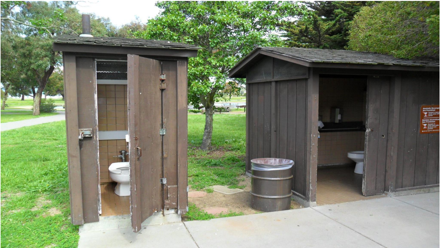
Photo 7. Before Project: Restrooms were in poor condition, could not keep up with demand, were often over crowded, had no sinks for handwashing, did not meet current health codes, and did not meet current ADA code. (Photo by Jeff Rasmussen)
