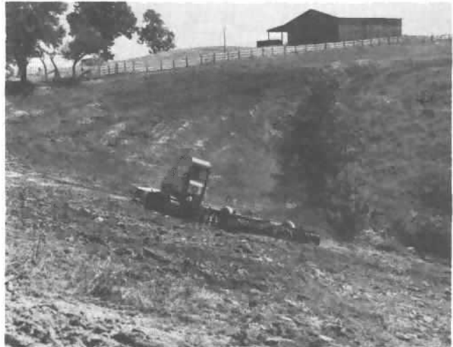
Breaking Up Excessive Compaction
