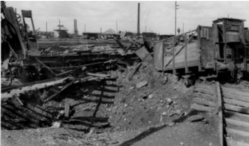
Wrecked rolling stock Hamm marshalling yard
