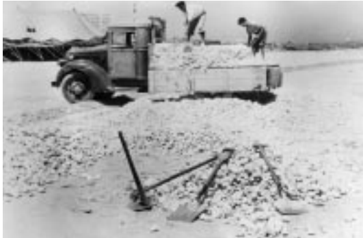
Maltese civilians repair airfield August 1942
