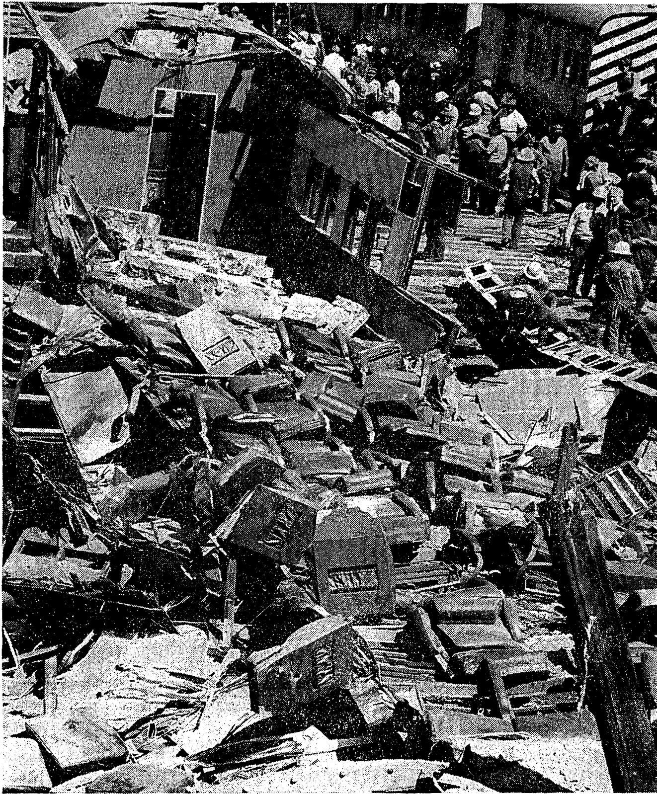
A mass of flattened seats was all that remained of a railway carriage when the last of the concrete slab that covered it was removed.
