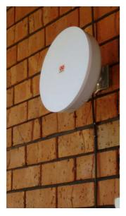
The size of domestic house bricks provide indication of relative size of dish and size of cable. Cable and clips will be similar colour to existing school external colour scheme.
