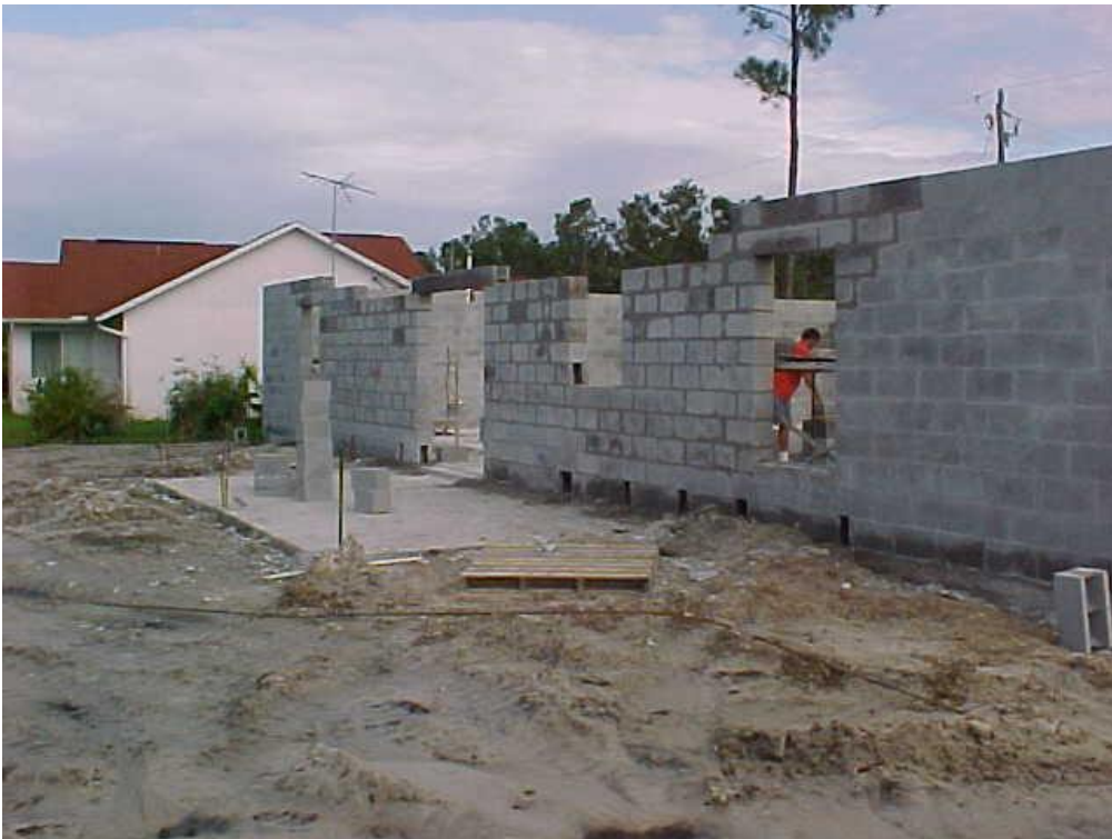
Photo -Rear Elevation
